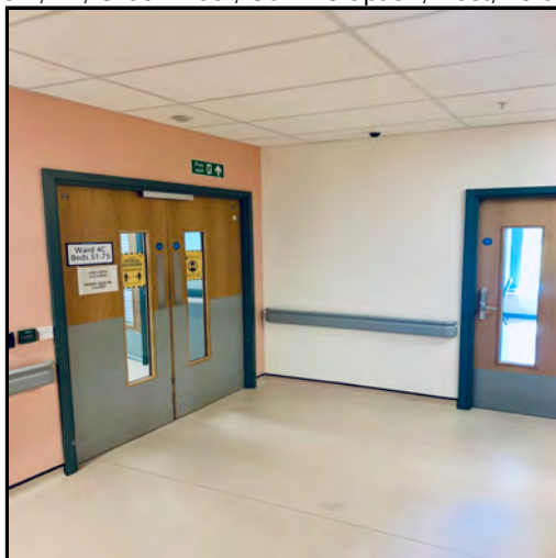
QEUH, L4, Green Roof, Access 5, Middle Door, 13 07 21
