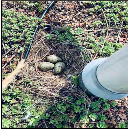
QEUH, L4, Green Roof, Gull Disruption, Nest, 13 07 21
