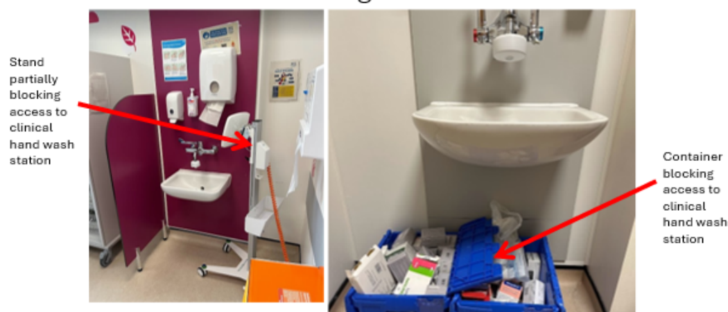
Figure 49. Storage of equipment and boxes that i) will prevent access to sinks and ii) will be splashed by contaminated water from the sink
