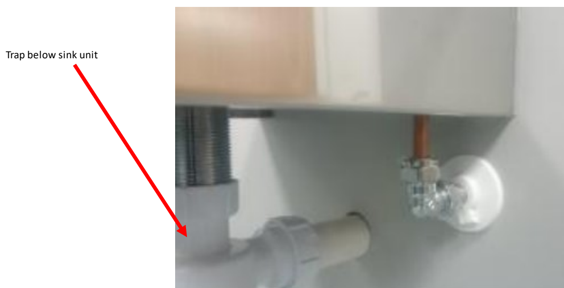
Figure 23. Position of trap below a sink unit.
