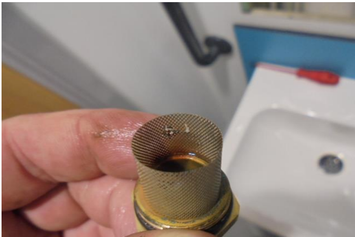
Minor Accumulation on Contour In-line Strainer
