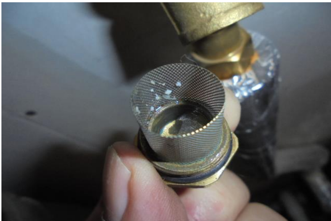
Installation Debris Retained in Contour In-line Strainer
