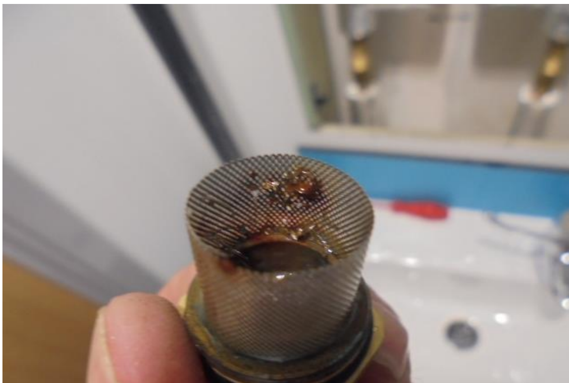
Substantial Debris Accumulation on Contour In-line Strainer
