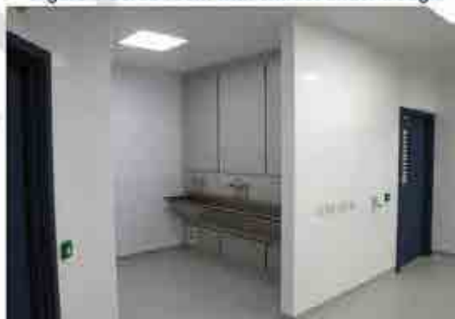
Figure 1 Scrub room with extract under trough
