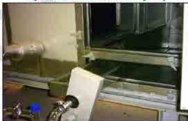
Figure 7 Removable AHU drainage tray
