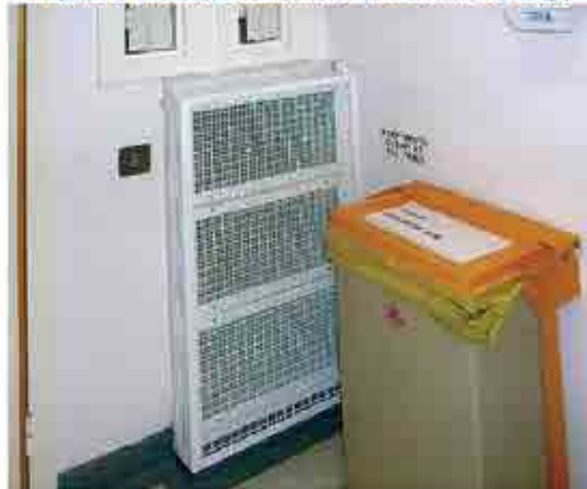
Figure 8 Pressure stabiliser with stand-off cage
