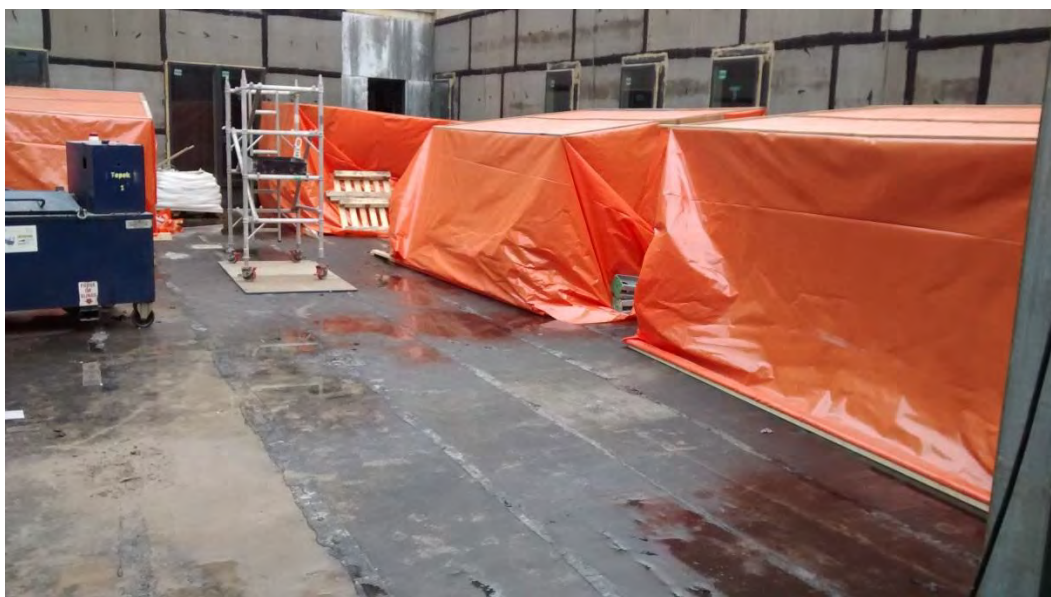
Fig 14 – Roof Waterproofing and Temporary Protection around Service Penetrations
