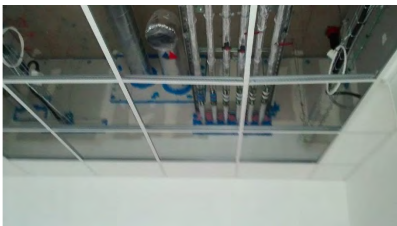
Fig 9 – Above ceiling Partition showing fire stopping of penetrations
