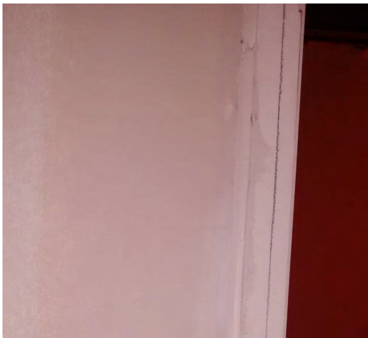
Figure 5 – Fire stopping seal around installed door frame
