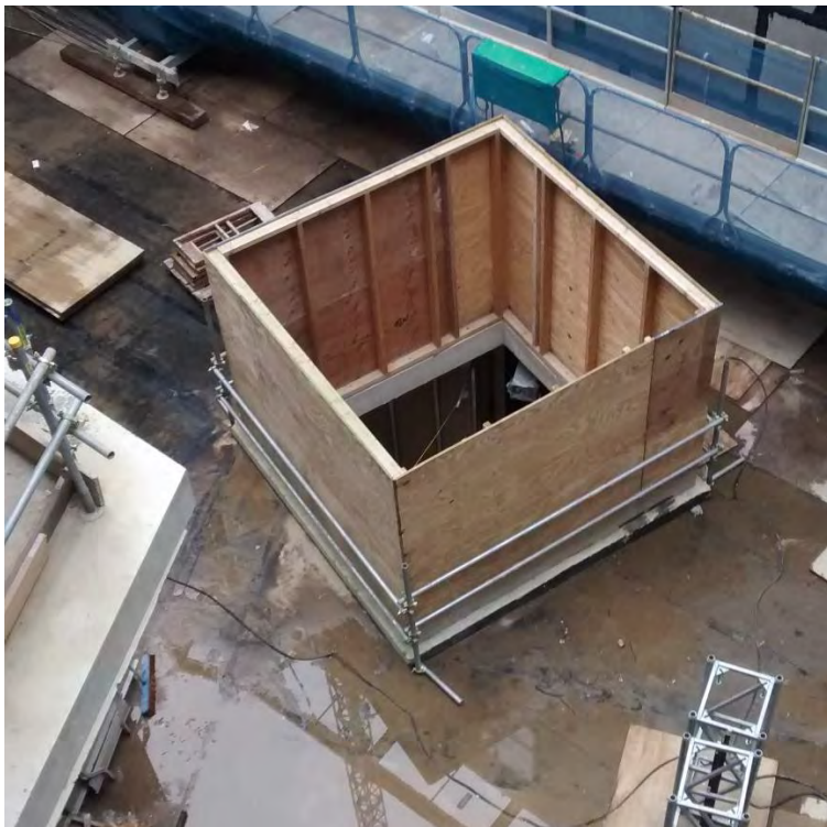
Fig 18 – Slab to be completed following removal of Tower Crane
