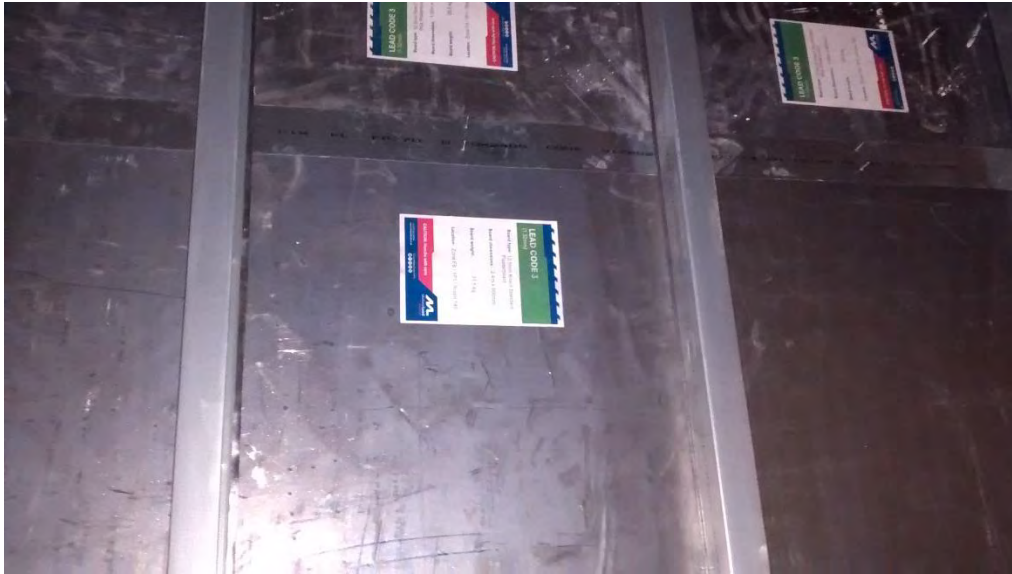
Fig 17 – Code 3 Lead Lining to Theatre Level 1
