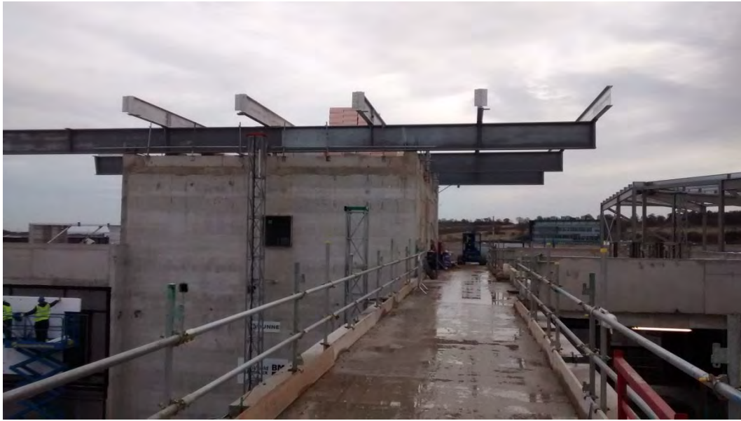
Fig 15 – Helipad Steelwork in progress
