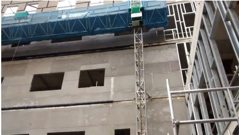
Figure 3 – Sealing of external boarding showing climber unit
