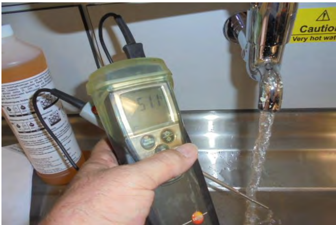
Hot Water Supply from Untempered Outlet Too Low
