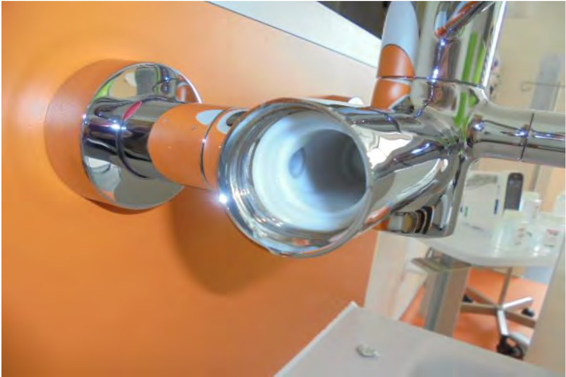
Hot and Cold Inlet Barrels to Markwik Thermostatic Taps Provided With Filter and NRV Cartridges
