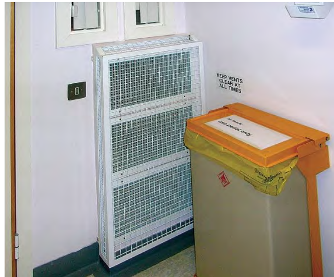
Figure 8 Pressure stabiliser with stand-off cage
