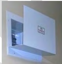
Figure 2 Pressure stabiliser fitted in preparation “lay up” room with stand-off baffle in theatre
