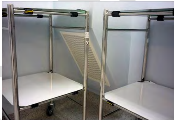
Figure A27 Low level extract recommended installation
