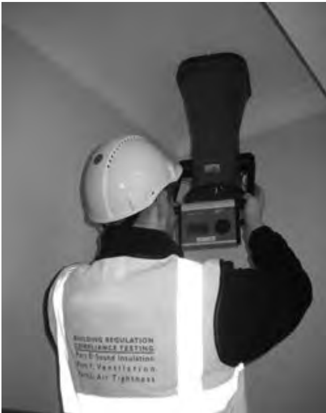
Figure 2.37 Flow hood (reproduced courtesy of BSRIA Compliance)
