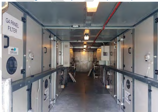
Figure 6 AHU plant room (internal)
