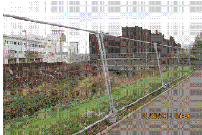
ON SITE FLOOD WORKS PROGRESS
