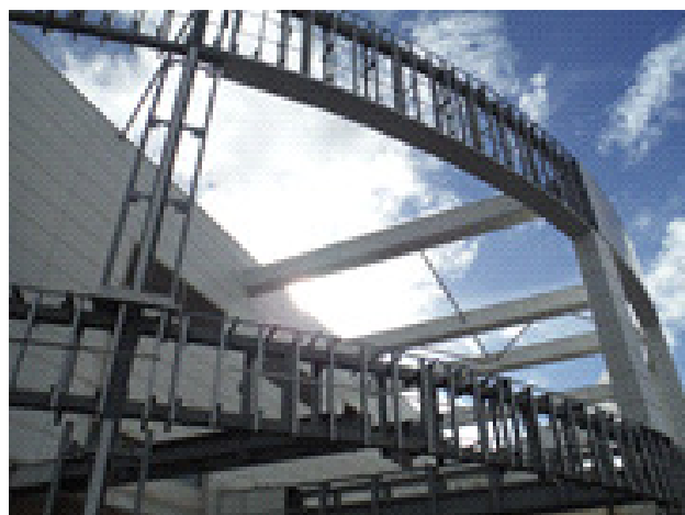
Part Drum Removal at RIE Emergency Department
